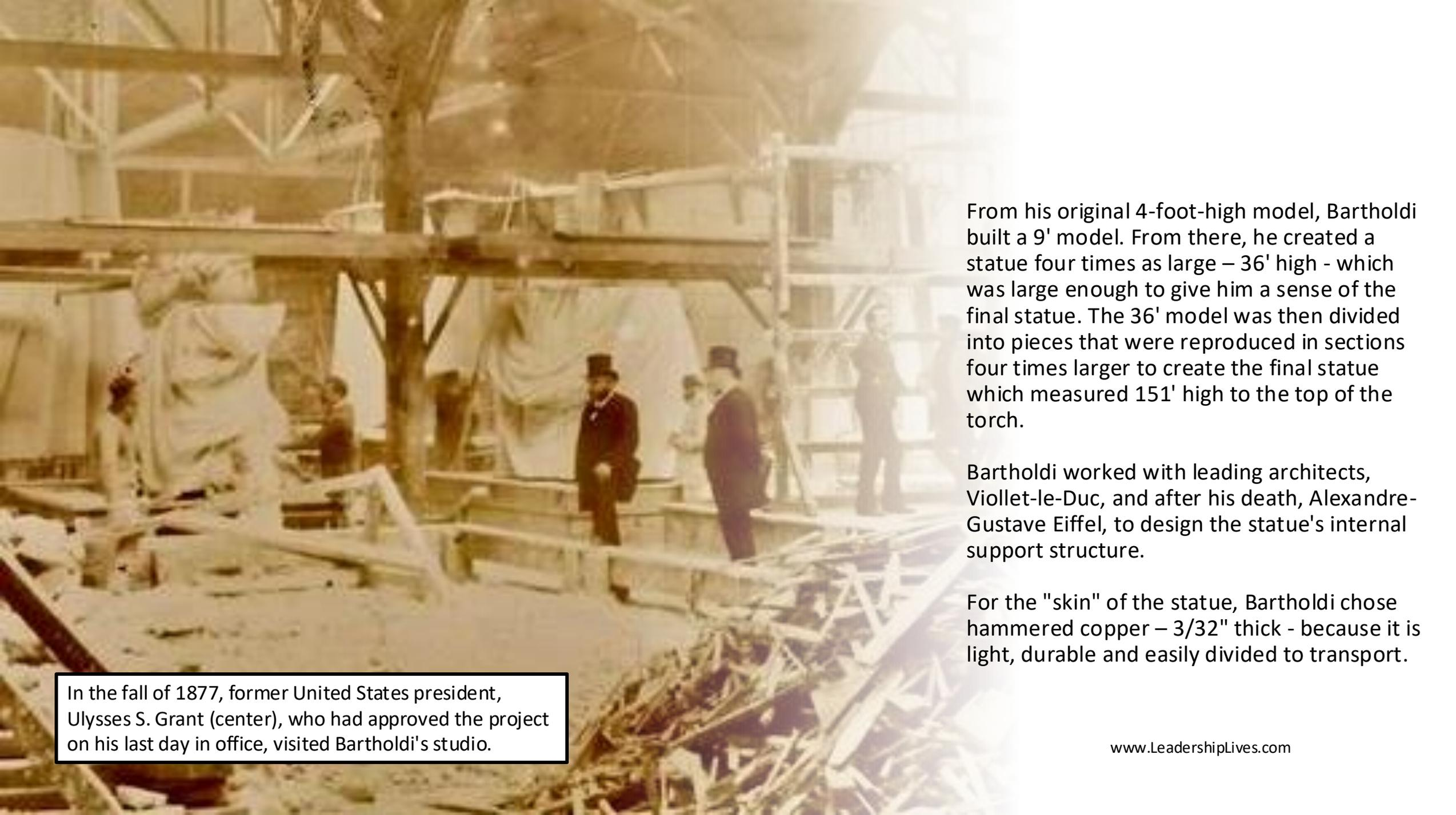
From his original 4-foot-high model, Bartholdi built a 9' model. From there, he created a statue four times as large – 36' high - which was large enough to give him a sense of the final statue. The 36' model was then divided into pieces that were reproduced in sections four times larger to create the final statue which measured 151' high to the top of the torch.
