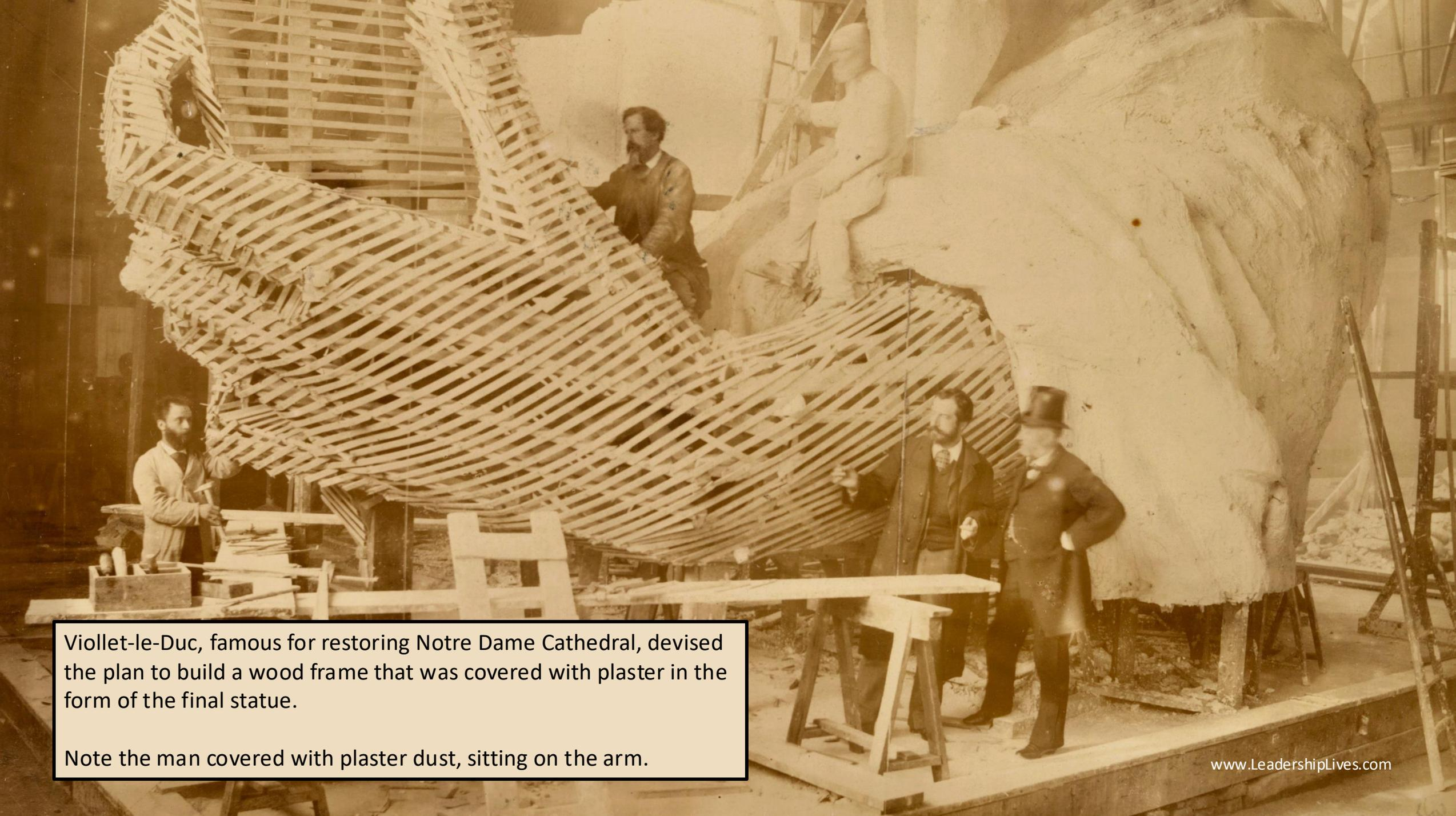
Viollet-le-Duc, famous for restoring Notre Dame Cathedral, devised the plan to build a wood frame that was covered with plaster in the form of the final statue.
